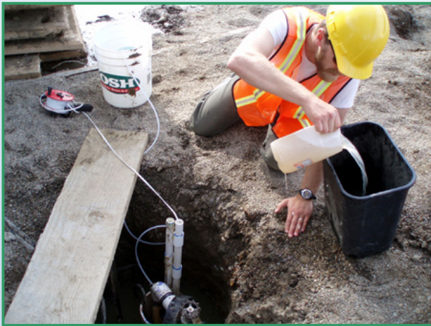
Measuring surface to groundwater depth
