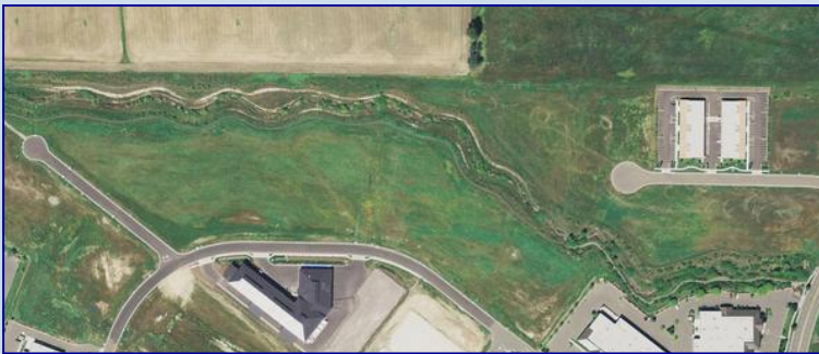
Restoration extends upstream and downstream from this central section of Sheehy Creek.
