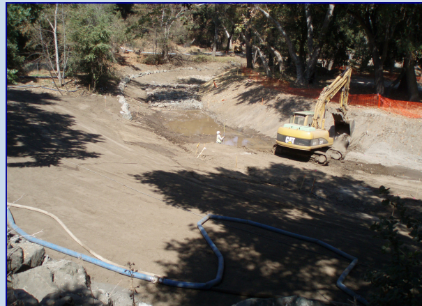
Construction of new stream
